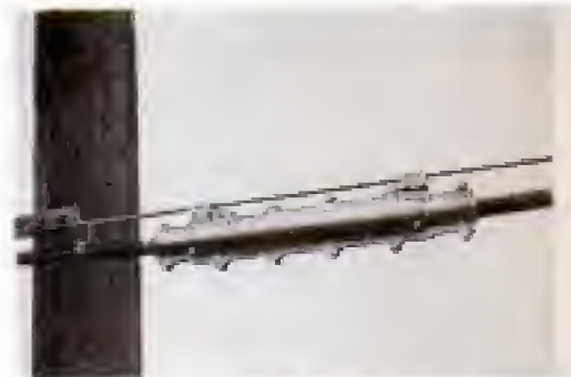
CLOSED CASING IN PLACE
